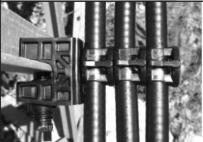
Maximum loading: 3 polymer hangers (shown) or two metal hangers.
