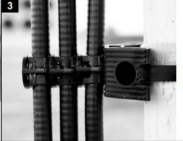
Configuration showing adapter securely attached to tower member.
