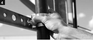
The front latches of the hanger should be squeezed to fit into the 34" hole.
