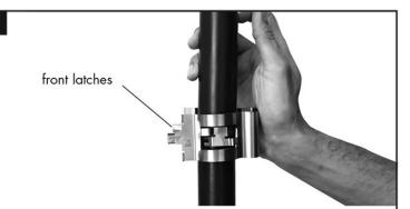
The installer might need to push the hanger onto the cable (away from the open end), to facilitate closing the front latches.
