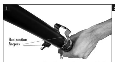
Position hanger onto the cable. Ensure four fingers of the flex section are on the cable. **NOTE: Make sure cable is straight.**
